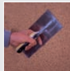
Application du Marbro Muro
